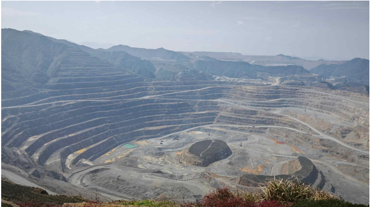
Jiangxi Group Dexing Copper mine.
